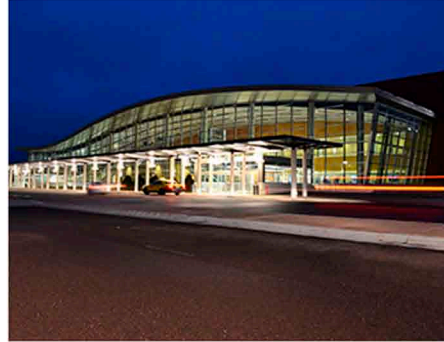
Duluth International Airport Reynolds, Smith & Hills
